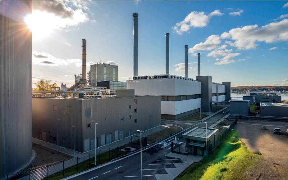
20 Jenbacher J920 Flextra gas engines make up the heart of the coastal power plant, generating 190 megawatts of electrical power for the German city of Kiel. "Photo Copyright -Stadtwerke Kiel"
